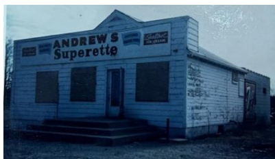
Andrews Superette became Apostolic Temple after serious renovation.
